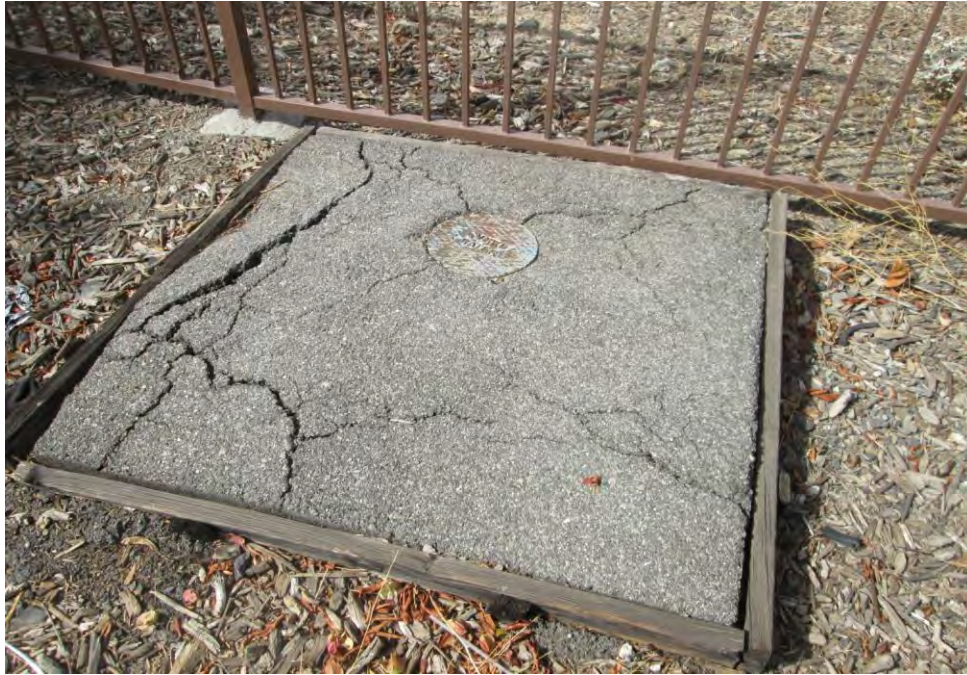
Water terminus at the Burnet Street cul-de-sac
